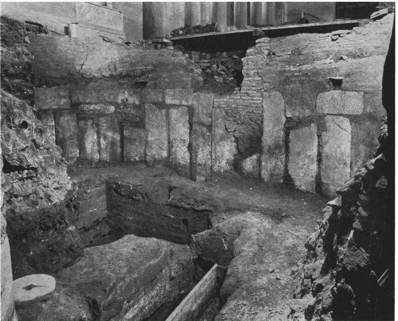
Fig. 60 — S. Lorenzo f.l.m. Excavations 1947-49. L-chamber, supporting pier, mensa oleorum , apse K , from northeast (Photo: Sansaini).
